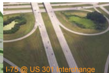
I-75 @ US 301 Interchange
